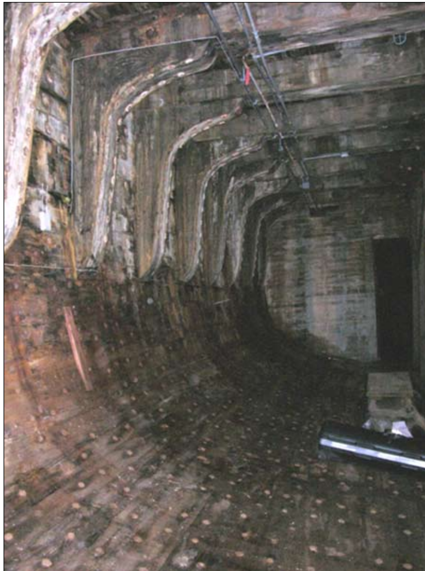
Aft view of main cargo hold showing ceilings, clamps, hanging knees, main deck beams
