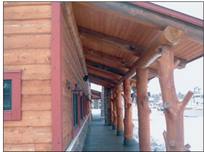
Rustic semi-structural application.
