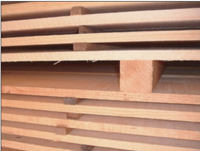
Figure 19—Misaligned stickers during drying result in warped lumber.
