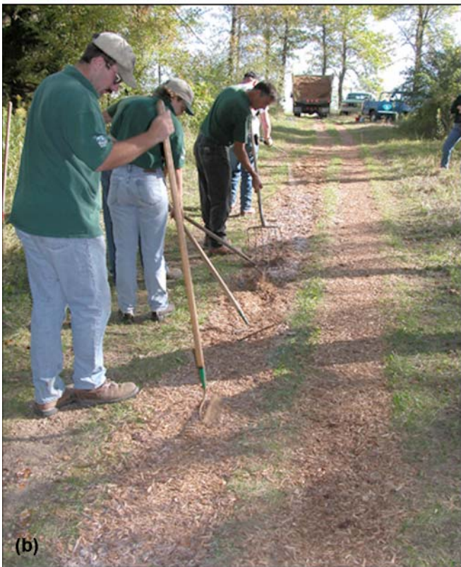
Figure 8—Installation of Soil-Sement surface on bridle path: (a) application of Soil-Sement by backpack-type sprayer; (b) trail crew mixed, leveled, and compacted the narrow trail filled with SEWF.
