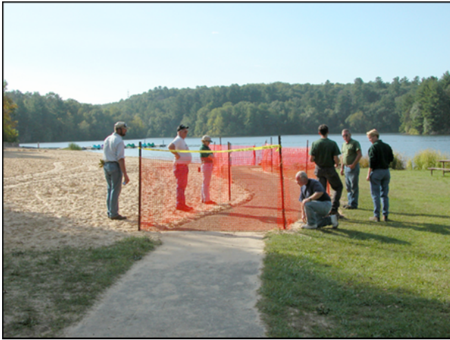
Figure 6—Completed beach path area looking west, shown with temporary barrier for 5-day SEWF curing period.
