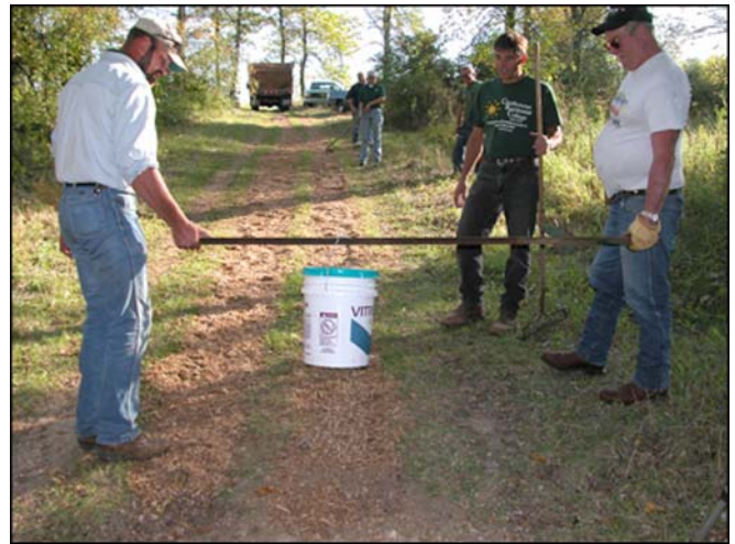
Figure 10—Application of Vitri-Turf to bridle trail by drip-bucket method. Holes drilled in bottom of 19-L (5-gal) container allowed uniform application over 0.4- by 20-m (1.3- by 66-ft) trail.
