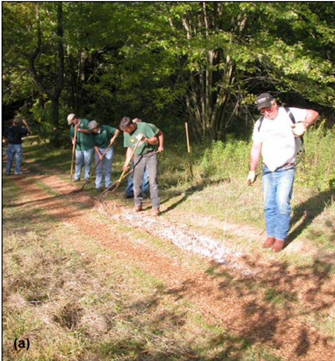
Figure 9—Application of Soil-Sement to bridle trail by drip-bucket method. Rakes were used to mix binder with EWF and level the trail.
