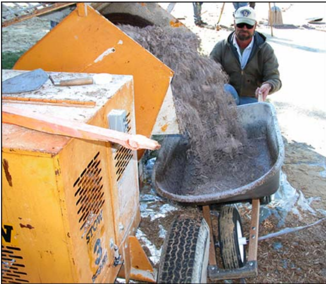
Figure 3—Loading of binder-EWF mixture from mortar mixer into wheelbarrow.
