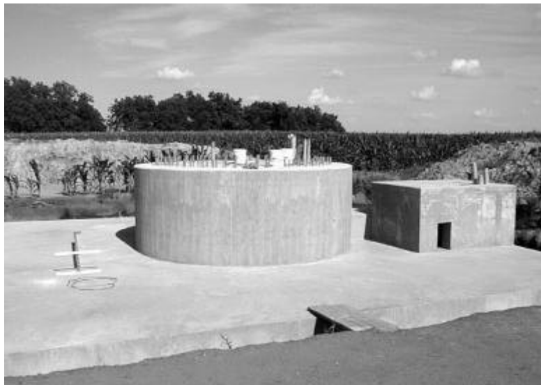
Figure 5. Inverted “T” Slab Foundation
