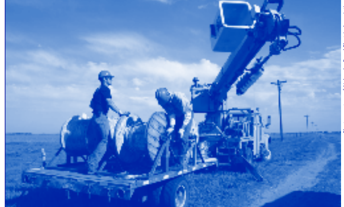
NVEMC Foreman Mark Thompson, center, changes a spool of wire with help from Shane Powell, left, and Steve Nelson, operating the digger truck.
