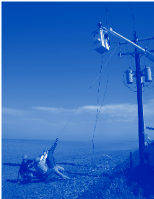
Lineman Jeremiah Krysl, in the bucket, connects the wire to the crossarm as the other crewmen remove the line sag.
