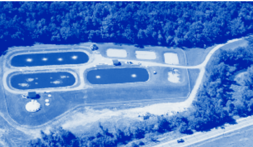
Carver, Minn. wastewater treatment facility
