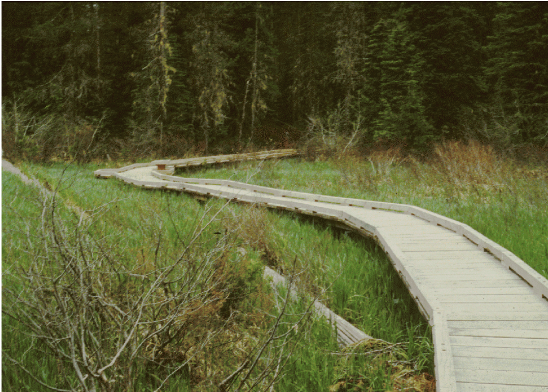
Figure 1—Wood treated with waterborne preservatives is often used for decking, such as in this wetland boardwalk.
