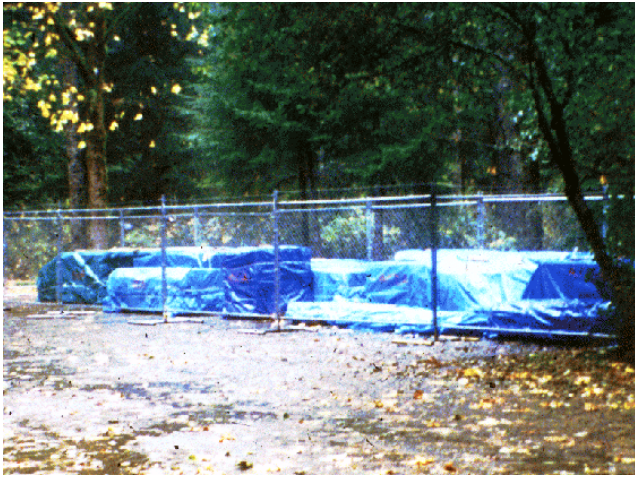
Figure 4—Treated lumber delivered for construction projects should be supported off the ground and covered.
