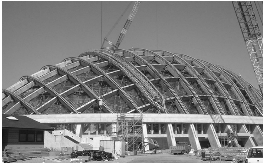
Fig. 10. Miyazaki-Dome built in 2004. Photo by S. Suzuki just after “the jack-down.”
