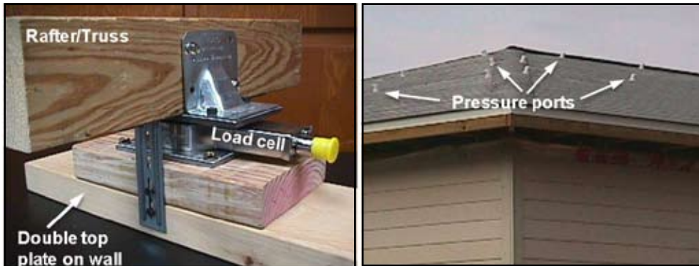
Typical instruments used on the roof of a test house.
