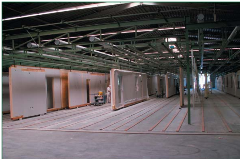
In a German modular home factory, drywall, wiring, doors, and windows are installed before wall sections are shipped to the construction site for assembly.
