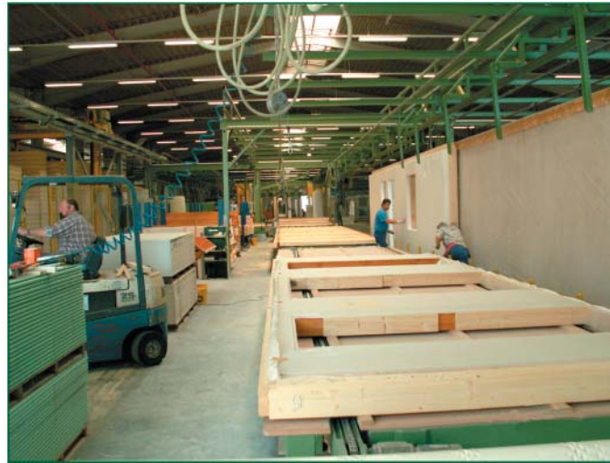
Wall sections progress down the assembly line in a German home manufacturing factory.
