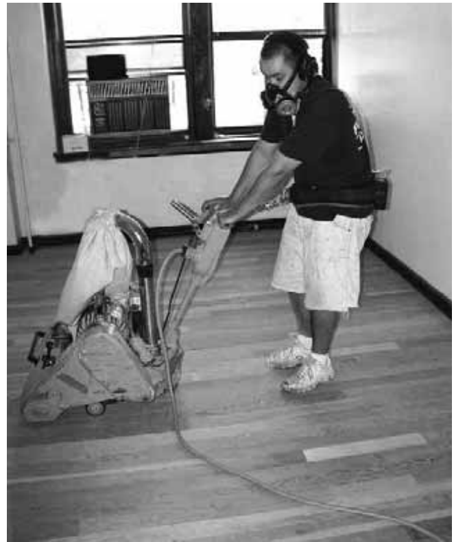
Figure 2. — Sanding of installed flooring. Note air monitoring pump on operator.
