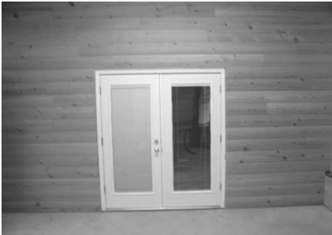
Figure 19—Log cabin siding on an interior wall section (7-in. width).
