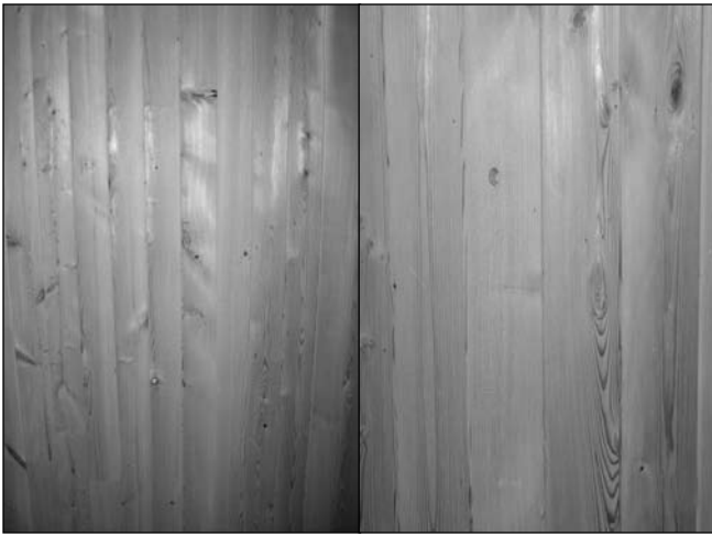
Figure 18—V-groove paneling of mixed grade qualities (left) and the higher C grade quality (right).
