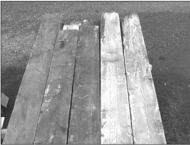
Figure 4 —Some lumber was clean, whereas other pieces had been painted or had surface contamination of cement or plaster.
