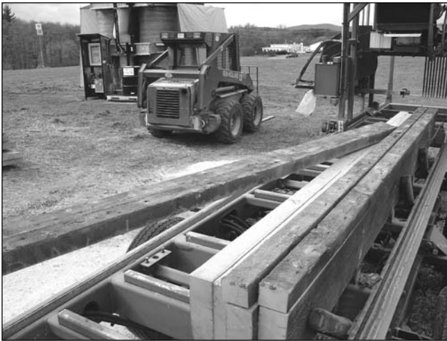
Figure 11—Edge sawing of 3 by 12 reclaimed hemlock. A 1-3/4-in.-depth cut was used to remove embedded edge nails.
