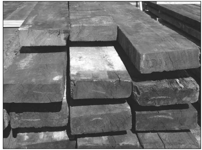
Figure 6 —The thickness of the lumber studied varied because it was originally installed rough sawn.
