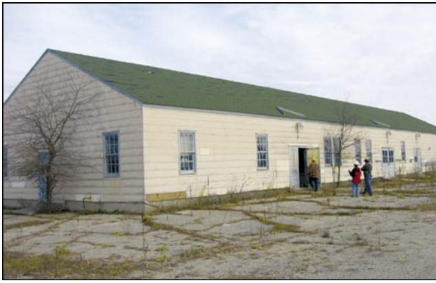
Figure 15—Type 10-6822 maintenance shop.
