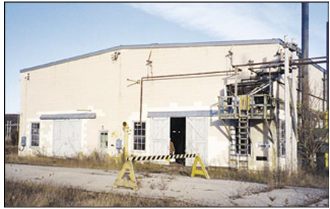
Figure 6—Type 4—700 compressor house.
