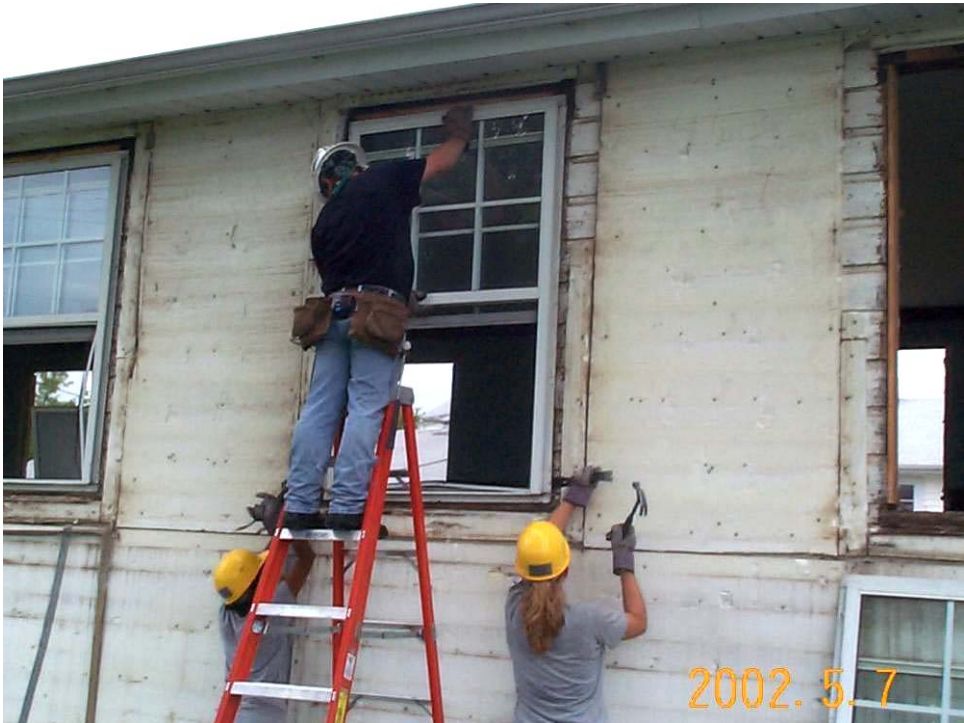
Figure 3. Deconstruction at Fort Campbell.
