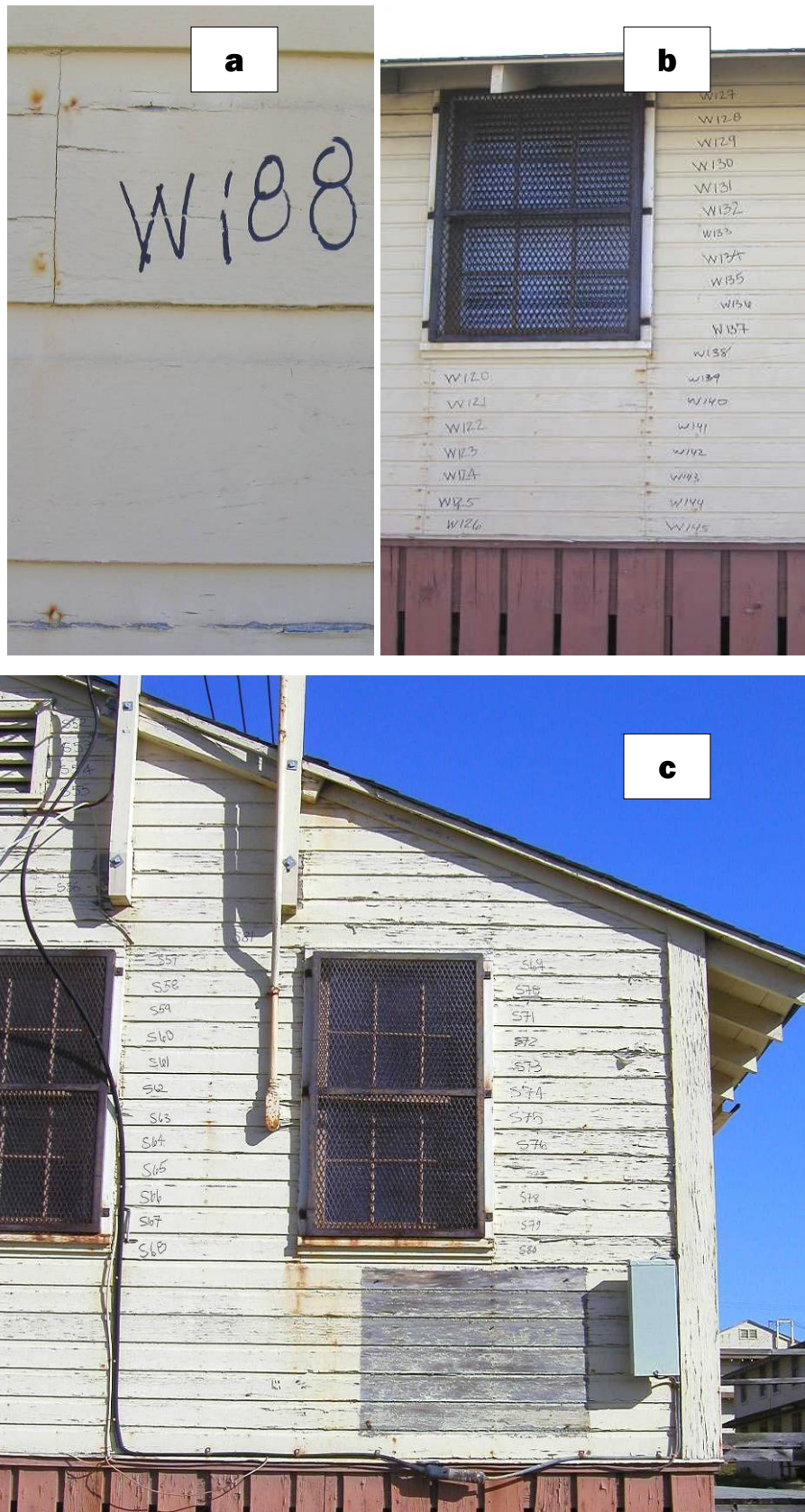
Figure 2. Typical ID numbering of individual siding pieces at Fort Ord.
