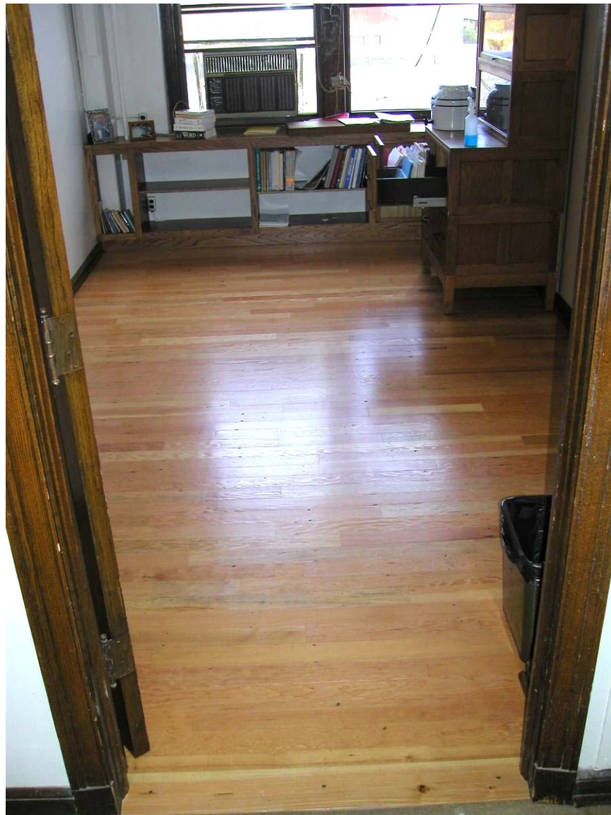
Figure 39. Installed floor after finishing.
