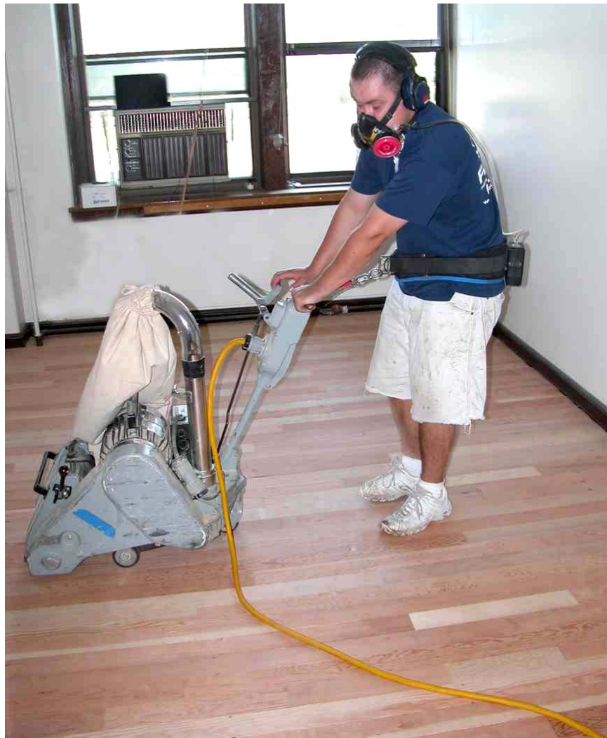
Figure 38. Sanding process for remanufactured flooring, showing air monitoring pump fitted at operator's waist.
