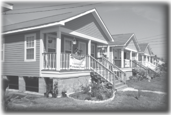
Houses with raised foundations recently constructed by Habitat for Humanity in New Orleans, Louisiana.
