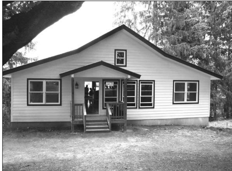
The completed HHFH home in Canton, NC.
