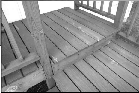
Finished Research Demonstration House decking.
