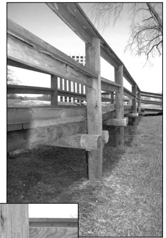
Properly connected joists and beams.
