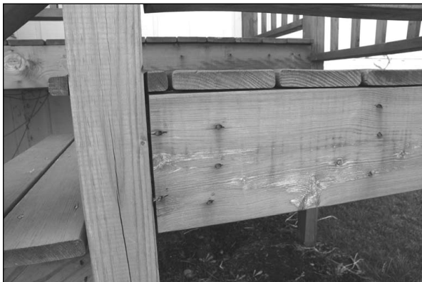
Spiral-groove or ring-shank nails are best used for decking.
