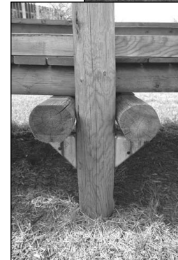
Properly connected joists and beams.
