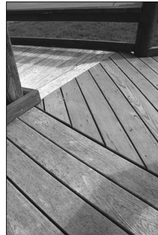
Research Demonstration House decking made using nine different preservative-treated woods, four wood-plastic composite materials, and three naturally decay-resistant species.
