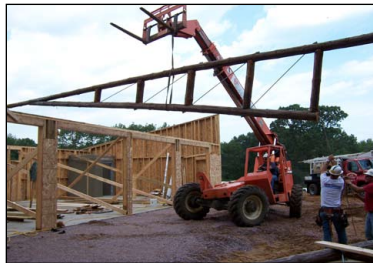
Raising the hand-peeled Leopold tree trusses.
