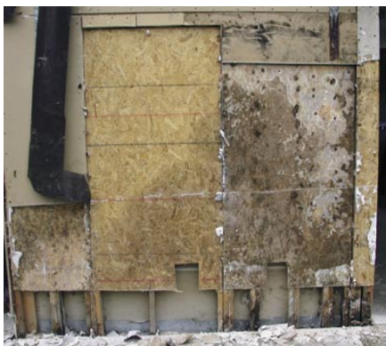
Top: Charlie Carll, forest products technologist, installs moisture monitoring equipment in the basement of FPL's Research Demonstration House. Bottom: OSB sheathing decayed from moisture accumulation under the siding of a condominium.
