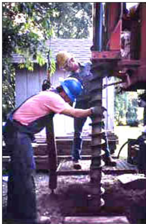
Al Wehrmann (left) and Bryan Coulson drill an observation well.
