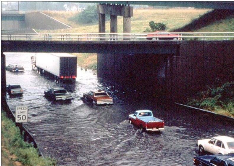
This flooded highway in East St. Louis after a heavy rainstorm resembles what would happen within minutes if the IDOT dewatering system failed.
