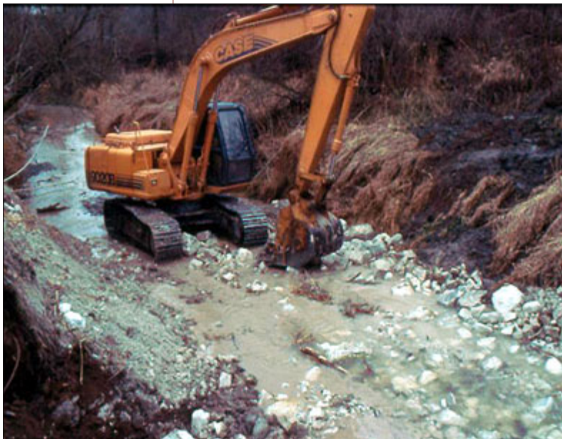
A riffle is constructed in the Spoon River watershed on North Creek.
