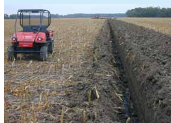
A new tile drain in northeastern Ohio.
