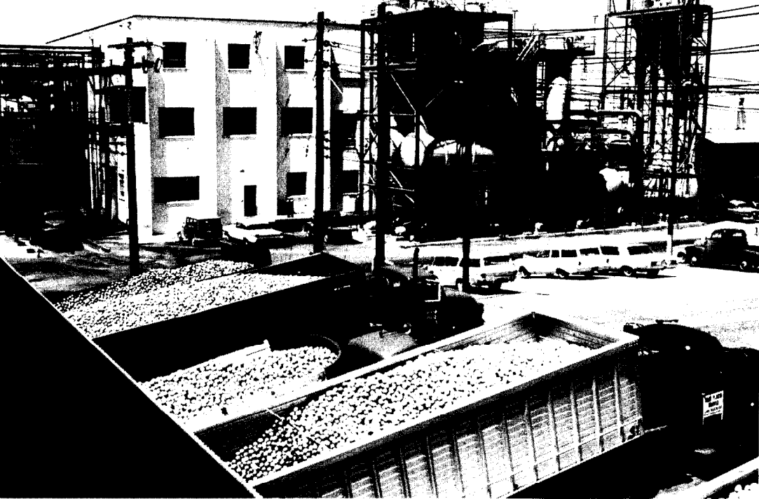
Florida citrus growers have made massive investments in facilities that process single strength juices, concentrates, sections, salads, dried pulp for cattle feed and by-products from oranges, grapefruit, and tangerines. This Citrus World plant is at Lake Wales, Fla.
