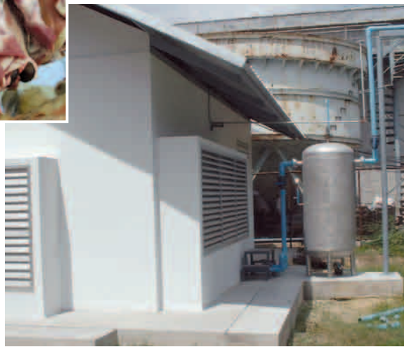
From abattoir to energy. A biodigester converts slaughterhouse waste into energy and solves two environmental problems—unhealthy waste and a need for power—at once.
