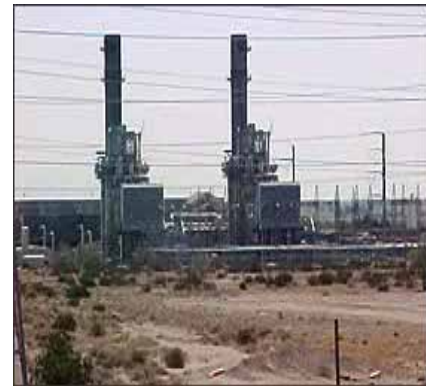
The same area after cleanup was completed.
