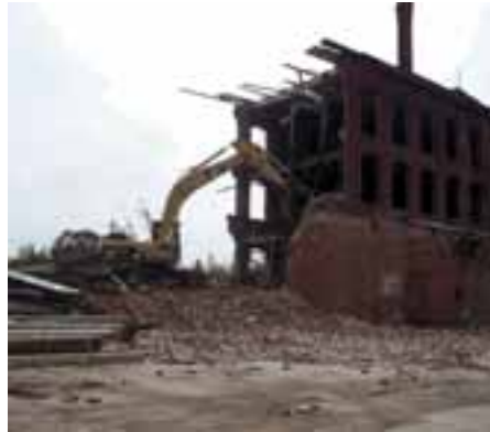
Manufacturing building being demolished as part of the Atlas Tack cleanup.
