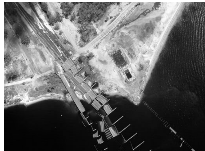
An image of a destroyed bridge on the east side of Biloxi, Miss. Credit: NASA
