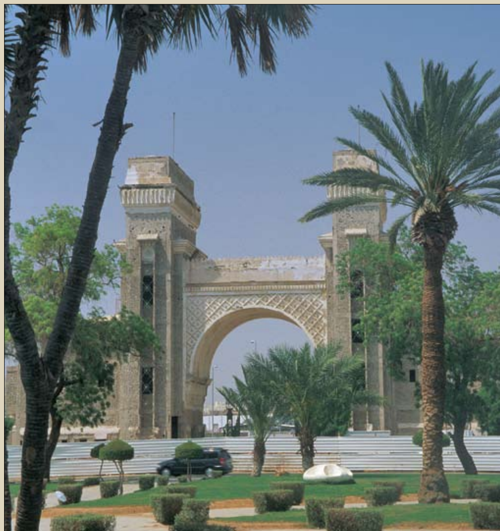
Mecca Gate, Jeddah
