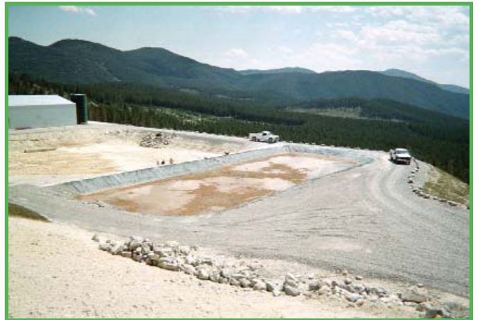
FIGURE 1. Sulfate-reducing bioreactor at the Luttrell Repository at the Basin Mining Area Superfund Site, Montana.
