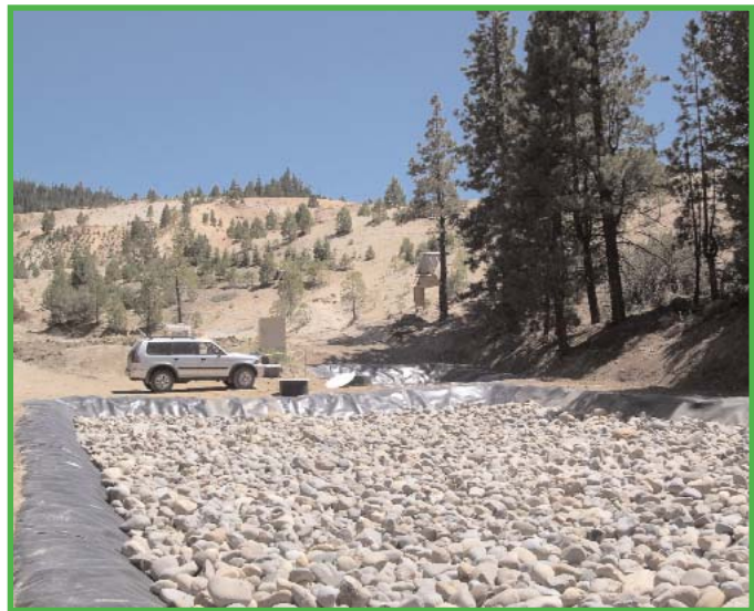
FIGURE 2. Compost-free “bugs on booze” sulfate-reducing bioreactor at the Leviathan Mine Superfund Site, California.
