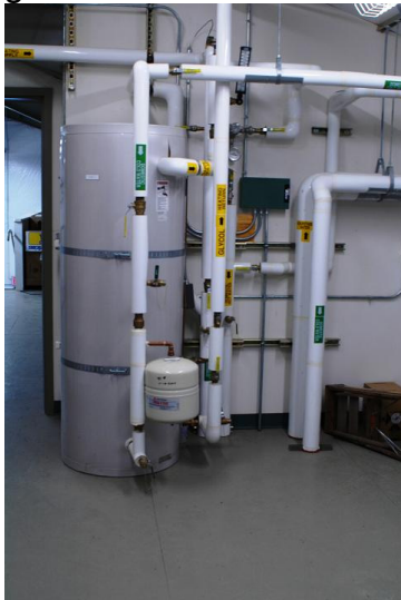
Kachemak McNeil Canyon Fire Station heating plant. Photo: Brian Saylor, March 10, 2008.
