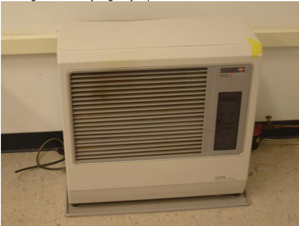
Toyostove heater in the multi-purpose room of the Tuluksak Youth and Multi-Purpose Facility, used to compensate for the building's inadequate heating system. Photo: Brian Yanity, March 5, 2008.
