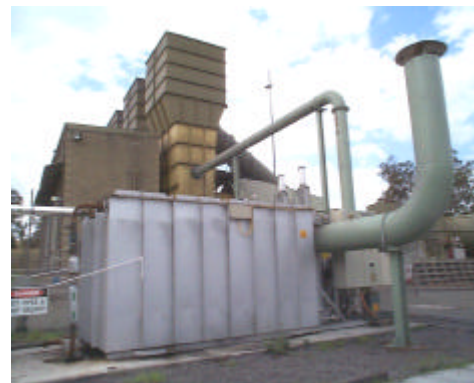
Vocsidizer Installation—Appin Colliery, NSW (Photo courtesy of BHP Billiton)
