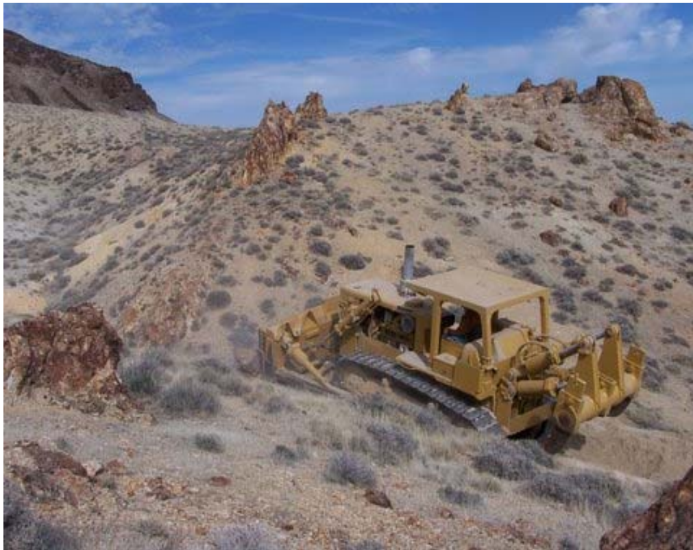
Notice-level access road building in Pershing County, Nevada
