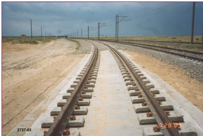
Figure 1. Independent Dual-Block Track (IDBT) at the demonstration site.
