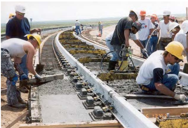
Figure 4. Construction of DFST Using Topdown Method
