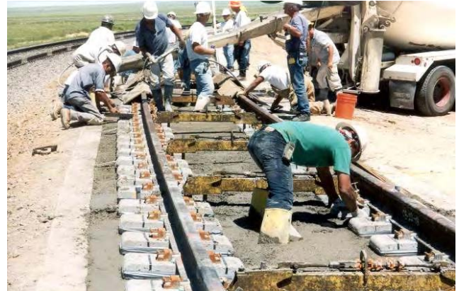
Figure 5. Construction of IDBT
