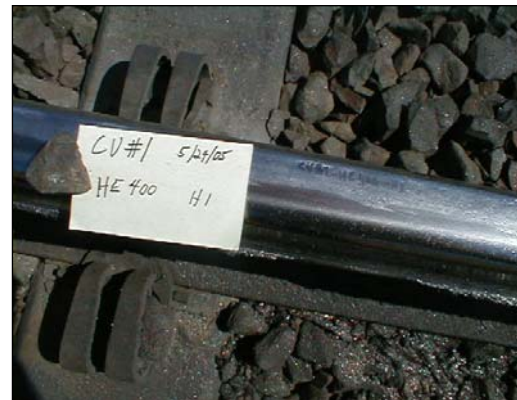
Figure 8. Photo of Rail Surface Condition After 169 MGT
