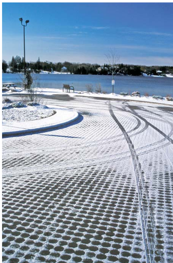
Breaking through barriers. Porous pavements come in many forms. Parking spaces in Columbus, Ohio (top left) are made of recycled clay aggregate. Shoppers at the Mall of Georgia, the largest mall in the U.S. Southeast, can park in a turf overflow lot (bottom left). The spaces between open-jointed pavers at Ontario's Sunset Beach Park lakefront access lot (above) admit water and prevent pollution of Lake Wilcox.
