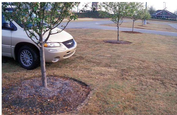
Breaking through barriers. Porous pavements come in many forms. Parking spaces in Columbus, Ohio (top left) are made of recycled clay aggregate. Shoppers at the Mall of Georgia, the largest mall in the U.S. Southeast, can park in a turf overflow lot (bottom left). The spaces between open-jointed pavers at Ontario's Sunset Beach Park lakefront access lot (above) admit water and prevent pollution of Lake Wilcox.
