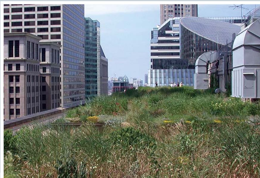
On top of the problem. The green roof atop Chicago City Hall contains more than 100 plant species that absorb stormwater and reduce the ambient air temperature by as much as 7–8°F compared to a nearby tar roof.
