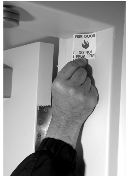
An example of the placement of the fire door stickers in the top corner on the hinge side of fire doors.
