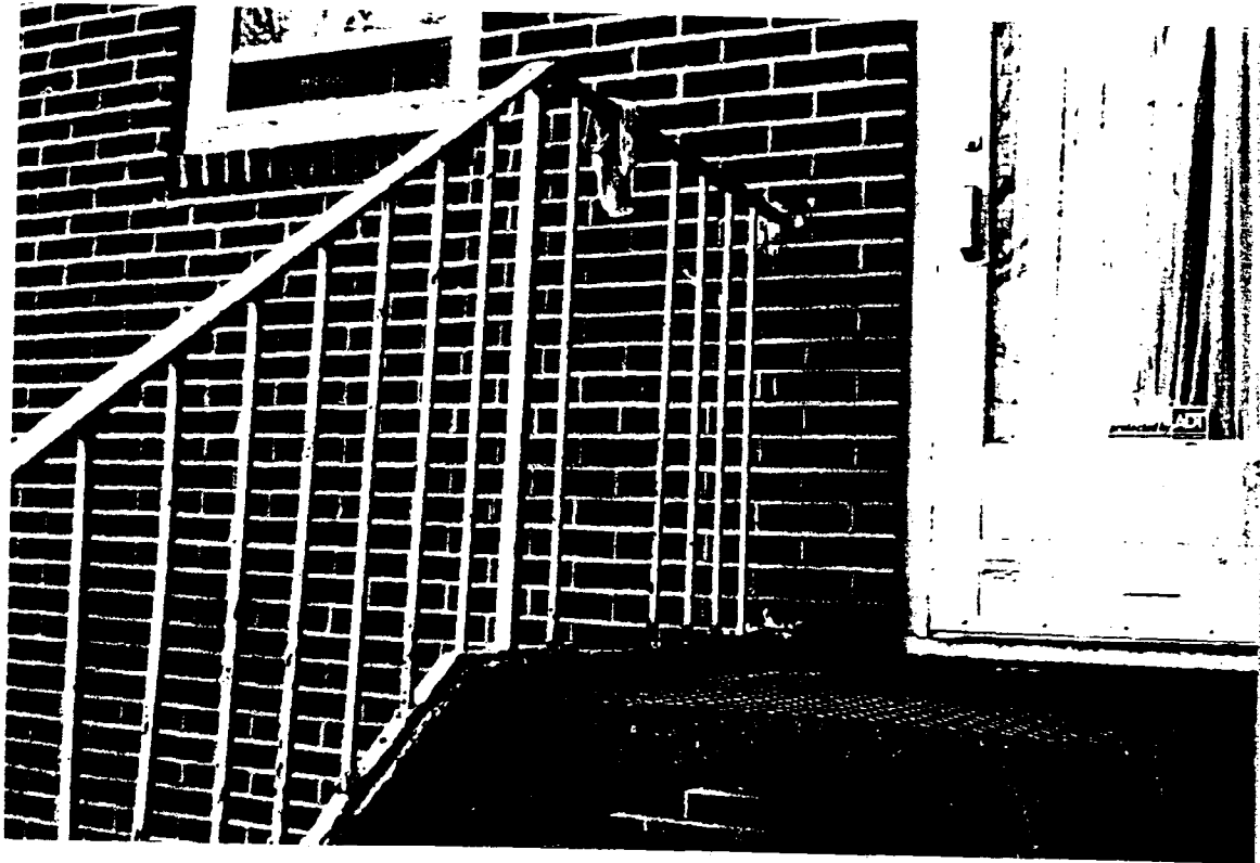
Deteriorating and unstable fire escape at foster care institution
