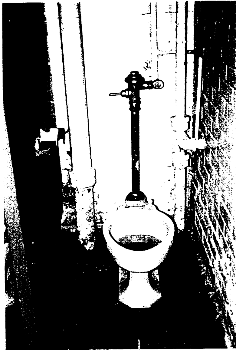
Unsanitary bathroom at foster care institution
