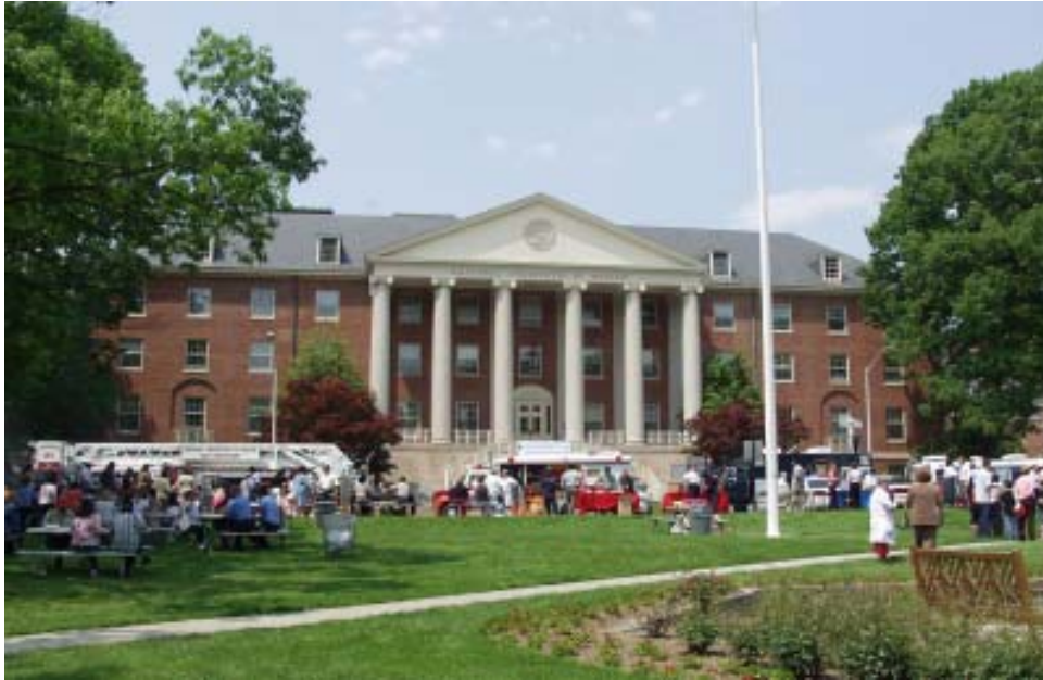
James A. Shannon Building
