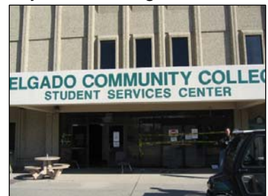
Repairs are in progress at the Delgado Community College.
