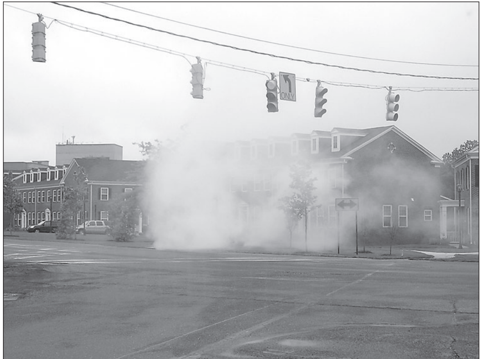
Figure 2: Steam Escaping from Pipes
