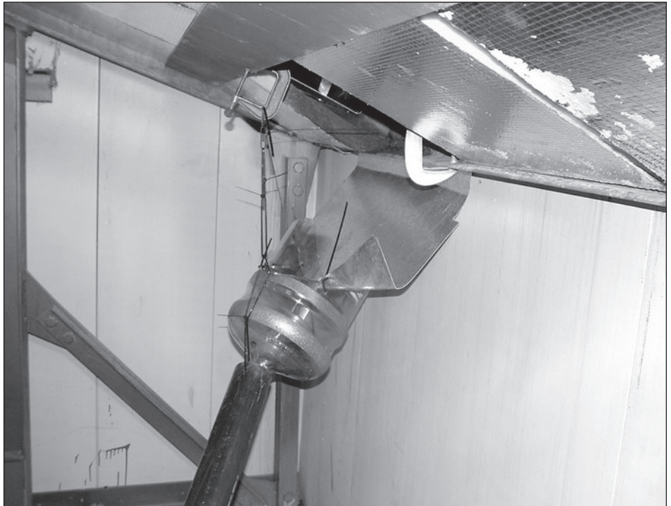
Figure 3: Roof Leak Drainage System
