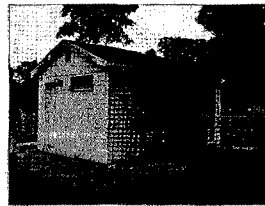
Deteriorated, Architecturally Incompatible Public Restroom Facility
