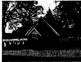
Deteriorated and Neglected Old Care Taker's House
