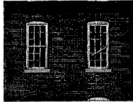
Historic Barn Deterioration
