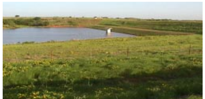
Sergeant Major Dam No. 2 after rehabilitation.
