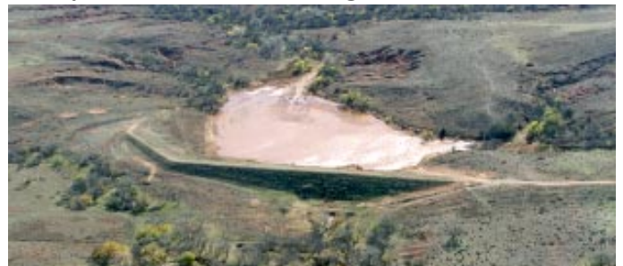
Sergeant Major Dam No. 2 before rehabilitation.
