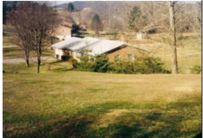
THE PROBLEMS. Development downstream requires upgrading the dam to meet safety criteria. Marrowbone Creek Watershed has protected homes, roads, bridges, farmland, and residents for almost 40 years.
