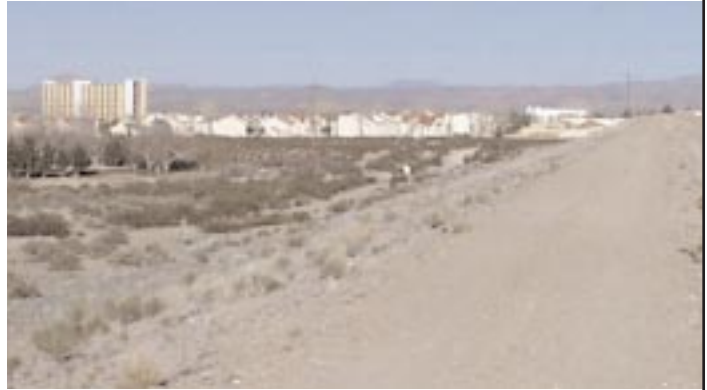
THE PROBLEMS. Downstream development has resulted in the need for the dams to be upgraded to meet current dam safety laws and ensure continued protection of the watershed and lives of people living and working downstream. This photo is taken from the top of the dam, Tortugas Site 1. The high rise building on the left edge of the photo is Memorial Medical Center.
