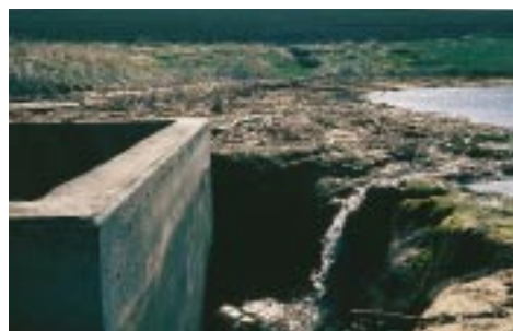
THE PROBLEMS. Dams filling with sediment (top) and deteriorating concrete spillways (above and left) are major, costly problems in the Little Beaver Subwatershed. Dozens of other dams face the same problems.
