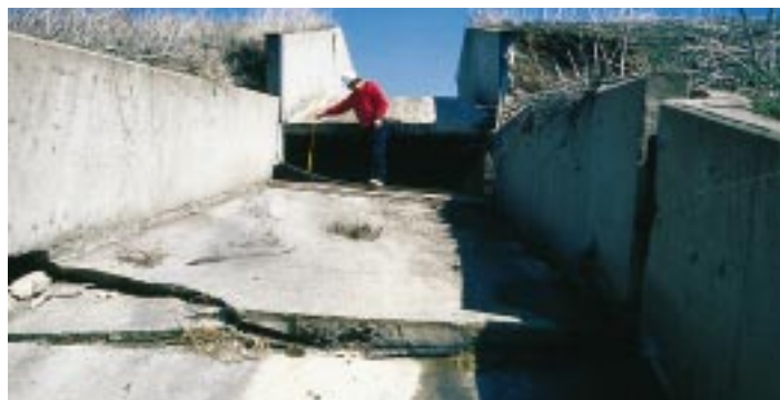
THE PROBLEMS. Dams filling with sediment (top) and deteriorating concrete spillways (above and left) are major, costly problems in the Little Beaver Subwatershed. Dozens of other dams face the same problems.
