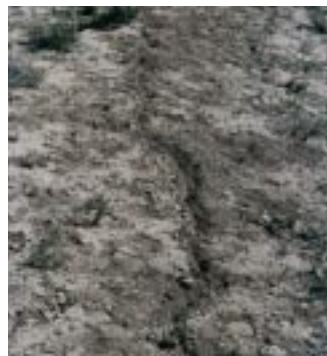
THE PROBLEMS. Top: Seep area below dam; note strong seep in gutter. Above: Cracks across dam (left) and above draw down pipe (right). In addition, the dams were constructed to protect agricultural lands, but downstream areas have since developed. This means the dams may need to be rebuilt, which will be costly.
