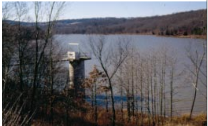
THE PROBLEMS. Concrete and steel in the main spillway will need repairs or replacement due to age (above). Houses and other buildings (left) were constructed below the dam after the lake was built. To meet today's dam safety laws, the dam will need to be rehabilitated.
