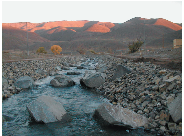
View looking upstream along the Derby Dam rock fishway.
