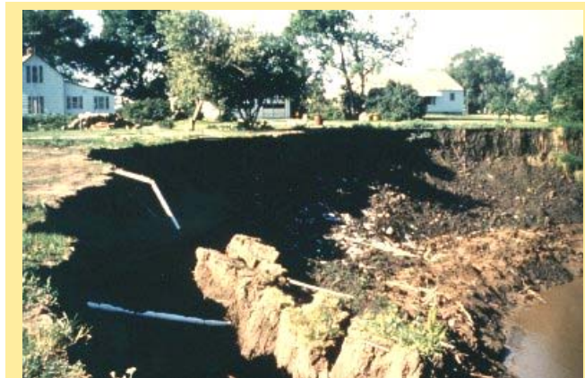
Fig. 1.1-1 Failed streambank threatens nearby homes
