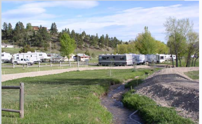
Now, the dikes on either side of the stream protect businesses and homes. The dikes have been lined with netting and seeded with grass to protect them from erosion.
