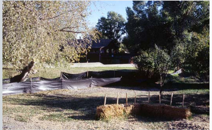
Above: Temporary barriers, like the sandbags, silt fence, and straw check dams above were used to protect homes from flooding prior to completion of the EWP project.
