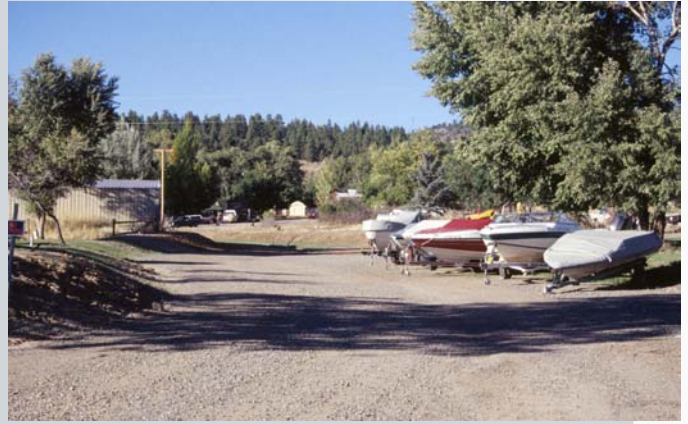
Some areas of rock armoring were needed in the channel to allow homeowners a safe, erosion resistant way to cross the stream channel to reach their homes. These boats are parked directly in the stream channel.
