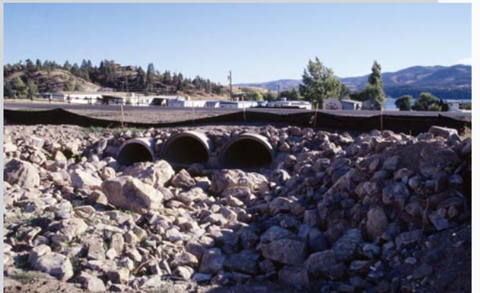
Now, the dikes on either side of the stream protect businesses and homes. The dikes have been lined with netting and seeded with grass to protect them from erosion.
