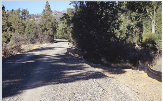
This access road to Forest Service, Bureau of Land Management, and private properties was built using the excess fill excavated from the channel. Construction was done and paid for by the Forest Service, BLM, and landowners.
