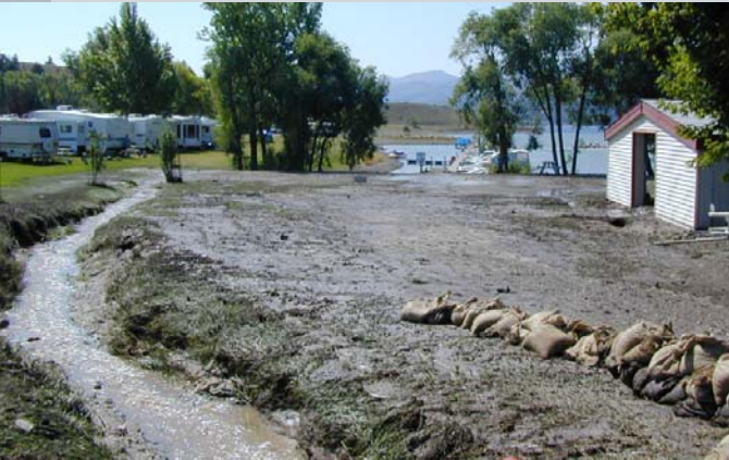
Before the dike and channel were constructed the flood waters ran into Kim's Marina.
