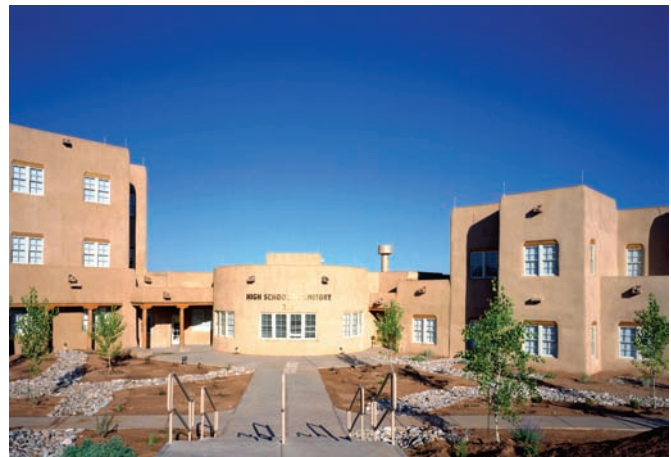
Santa Fe Indian School in New Mexico. A new $40 million, 250,000 sq. ft. campus with modern classrooms and dormitories for 900 7-to-12th graders has replaced buildings more than 100 years old. Approximately 60 percent of the students live on campus. The classrooms and dorms were finished in August, and a student life center is nearing completion.
