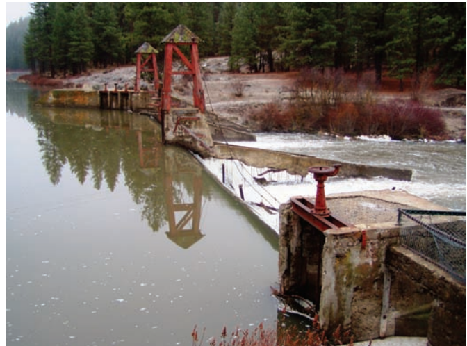
Removing the aging and dilapidated Chiloquin Dam will open up many miles of spawning habitat to endangered fish. Installing pumps will allow irrigators to continue to get the water once provided by the dam.
